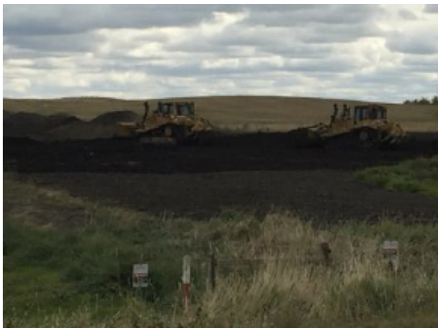
Dozer spreading seconds – SF 26 - Sept 28, 2018
