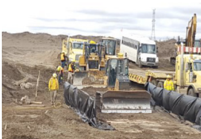
Rough cleaning equipment - SF 34 - Sept 29, 2018
