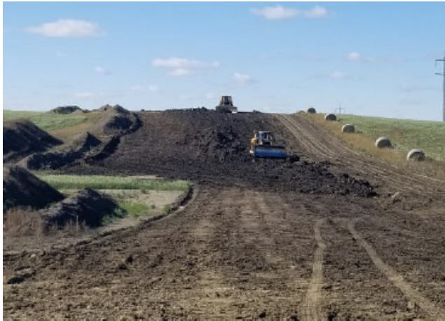
Dozer shaping and contouring – SF 40 – Sept 27, 2018
