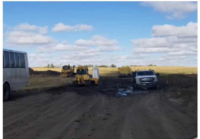
Water pumping at access – SF 27, Sept 27, 2018
