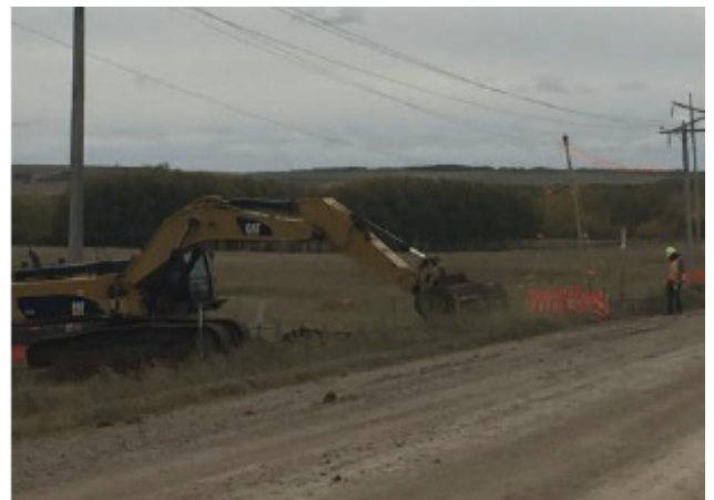
Excavators bailing out soil to dozers – km 56+000 - Sept 26, 2018
