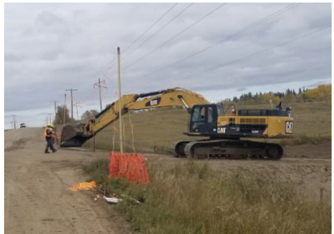
Excavator narrowing access ramp – SF 35 – Sept 28, 2018
