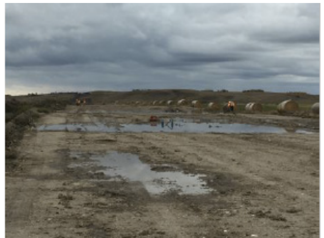
Utility crew pumping surface water – SF 28 – Sept 28, 2018
