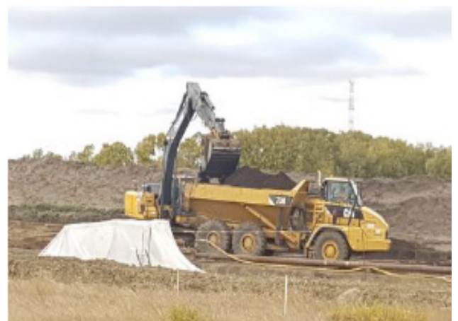
Excavator loading soil onto haul truck – SF 34 – Sept 29, 2018
