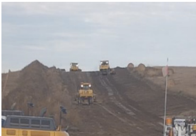
Dozer spreading topsoil and excavator working on roach – Sept 27, 2018
