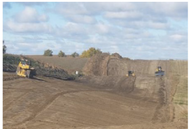
Dozer decompacting and shaping – km 58+200 – Sept 27, 2018
