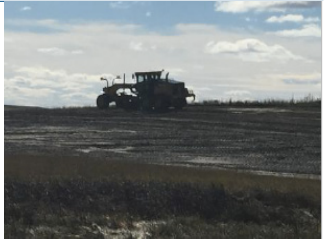
Grader shaping subsoil – SF 36 - Sept 27, 2018
